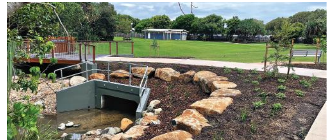
The park has had extensive drainage works completed along with new exercise equipment, BBQs and paths. Photo: Contributed
